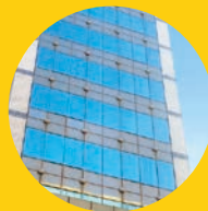
Java Road 108 Commercial Centre
