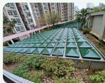
Waterproofing at SSC
