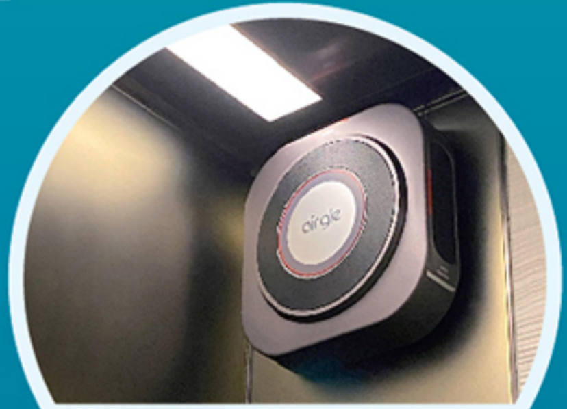
Air purifiers with HEPA filters and UV modules are installed in all lift cars of Dah Sing Financial Centre
